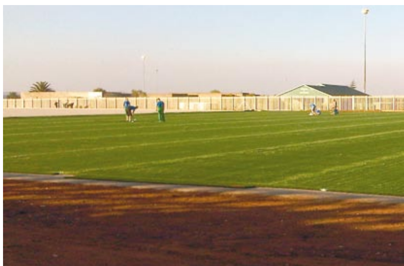
Adding the finishing touches
